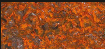
Without corrosion protection treatment
